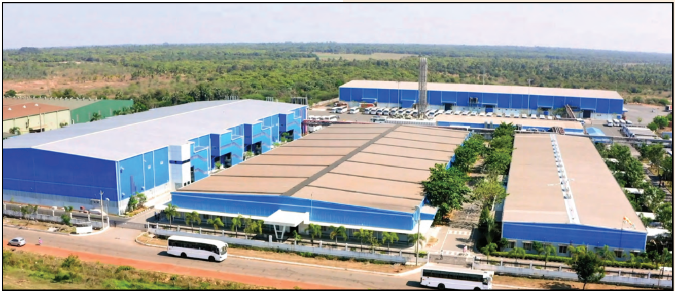
The world's largest mobile phones manufacturer Foxconn's manufacturing plant in Sri City
